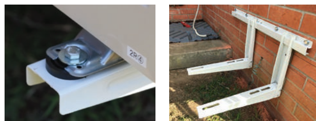
Figure 5: Wall mounting brackets
